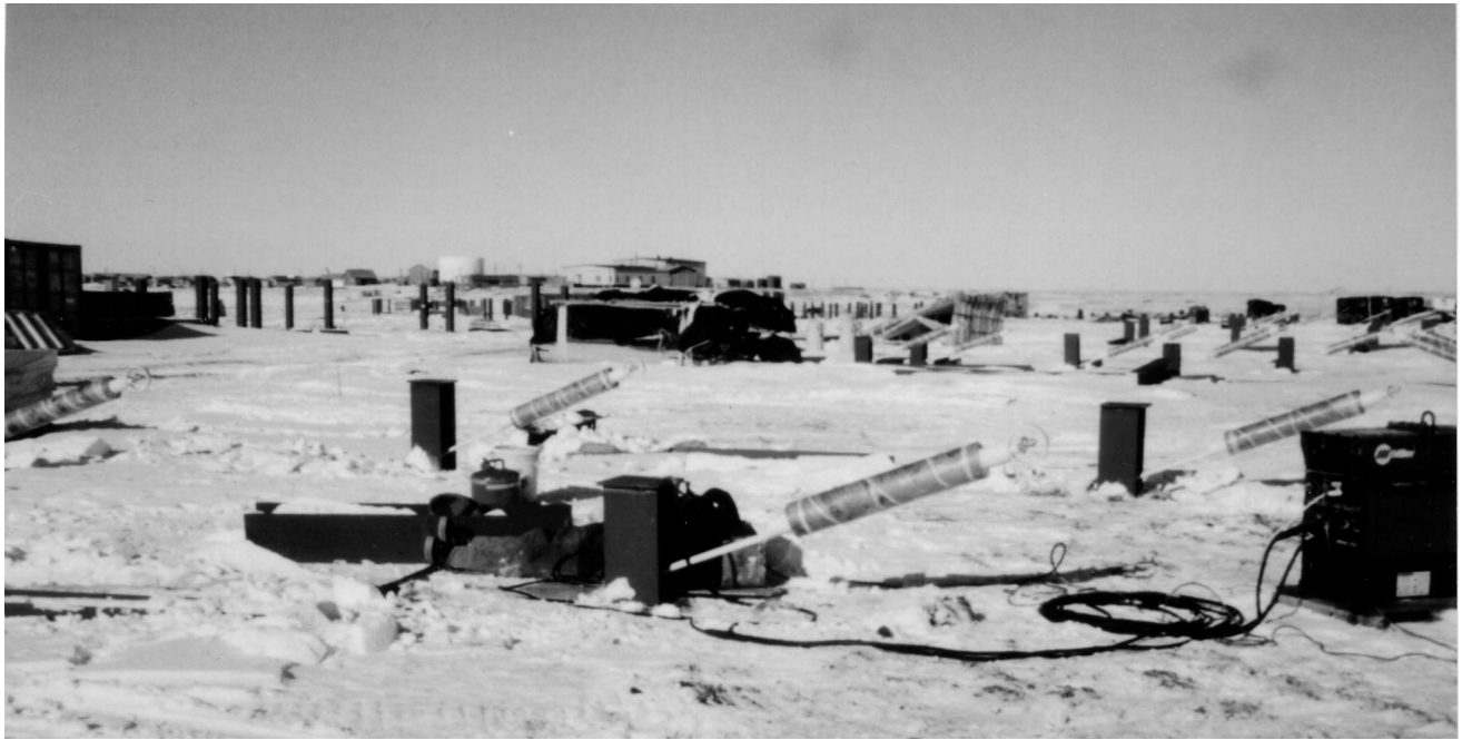
Figure 4. Installed Heat Tubes in H-Piles, Kongiganak Project Site.
