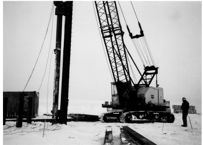
Figure 3. Installation of H-Piles, showing Crane and Hammer, Kongiganak Project
