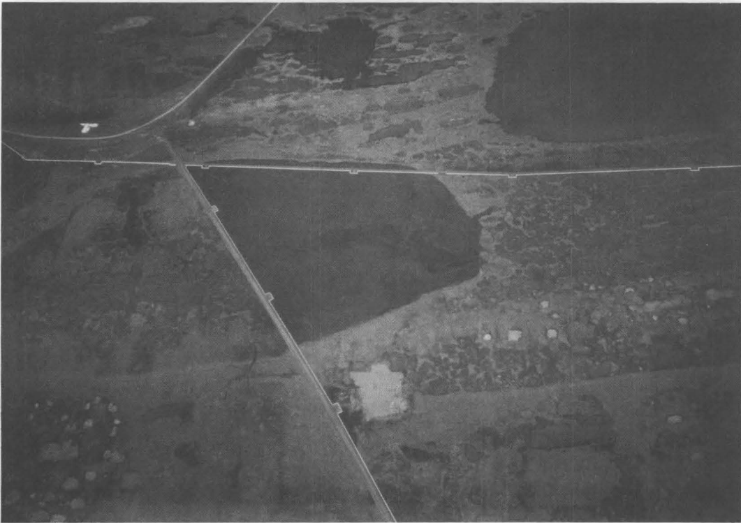
Plate 17. Impoundment caused by gravel road blocking sheet drainage across an old lake basin. Pipeline parallels the road.
