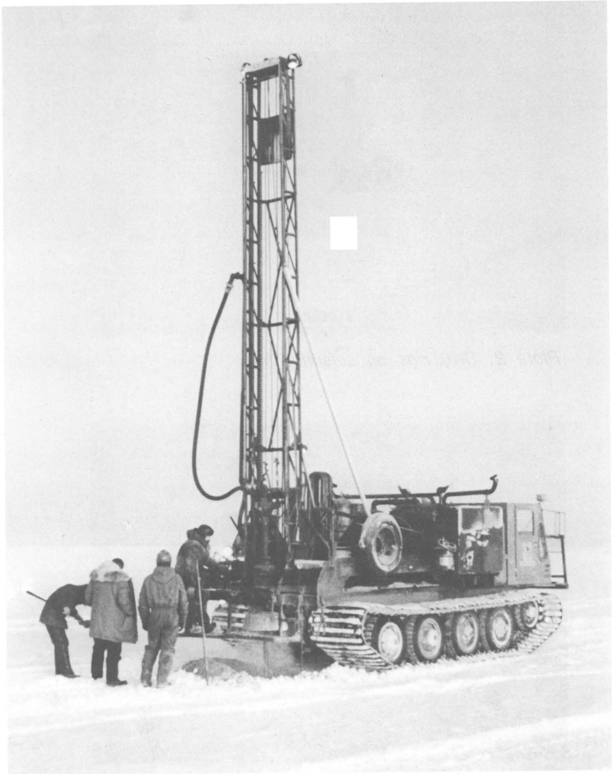
Plate 1. Mobile drill rig drilling shothole in which to place dynamite.
