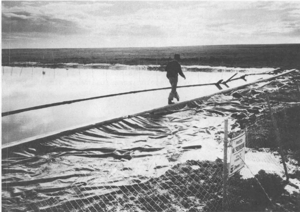
Plate 20. Plastic-lined reserve pit adjacent to the Chevron exploratory well, near Barter Island.
