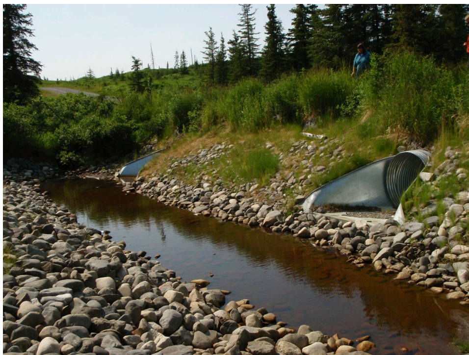
Figure 14. Culvert replacement with relief pipe on NNA1047.
