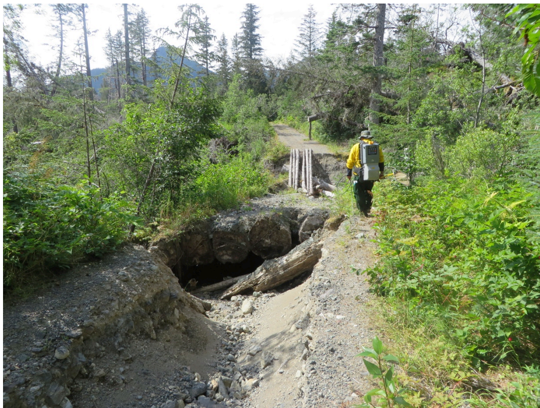
Figure 17. Collapsed log stringer bridge on Stream No. 242-32-10160 (Bridge 157 on Figure 11 map)
