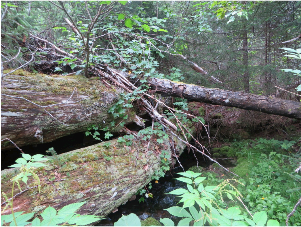
Figure 18. Failing log stringer bridge on Stream No. 241-11-10740 (Bridge 219 on Figure 10).
