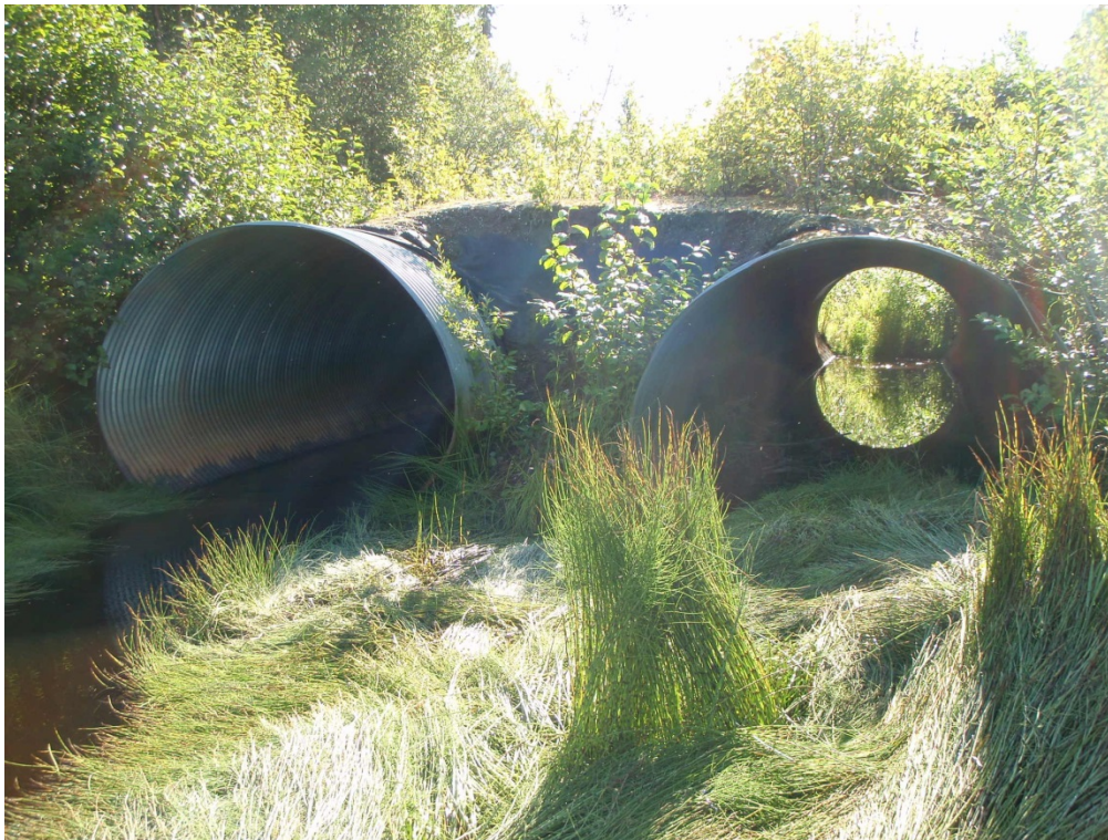
Figure 13. Twin culverts with a rating of 4, Tyonek.
