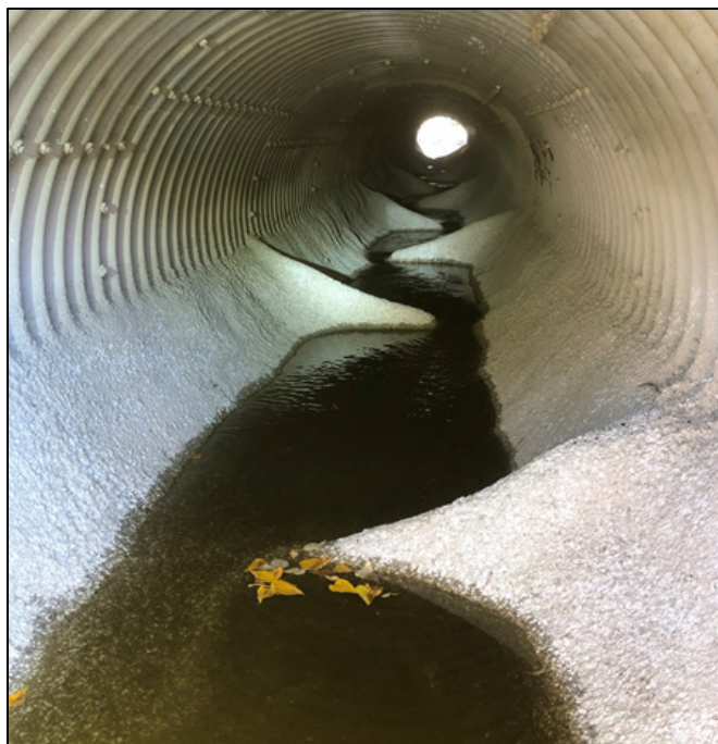
Figure 1. Culvert with rounded baffle design.
