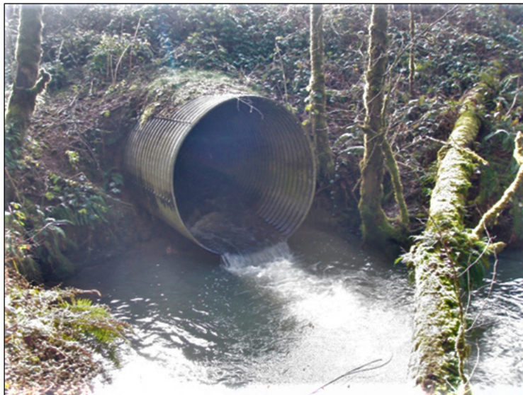
Figure 1. Pass Creek pre-retrofit, showing undersized culvert with perched outlet.
