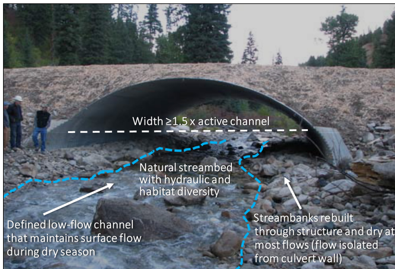
Figure 9. Example of a culvert replacement built with stream simulation design elements, Roaring River, Idaho. Credit: USDA Forest Service.
