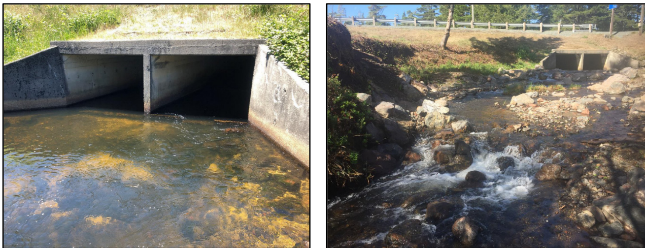
Figure 2. Post- project photos showing the modified baffle at culvert outlet and increased elevation of the outlet pool providing continuous passage into the culvert without requiring a jump (left) and the roughened channel downstream of the culvert (right).
