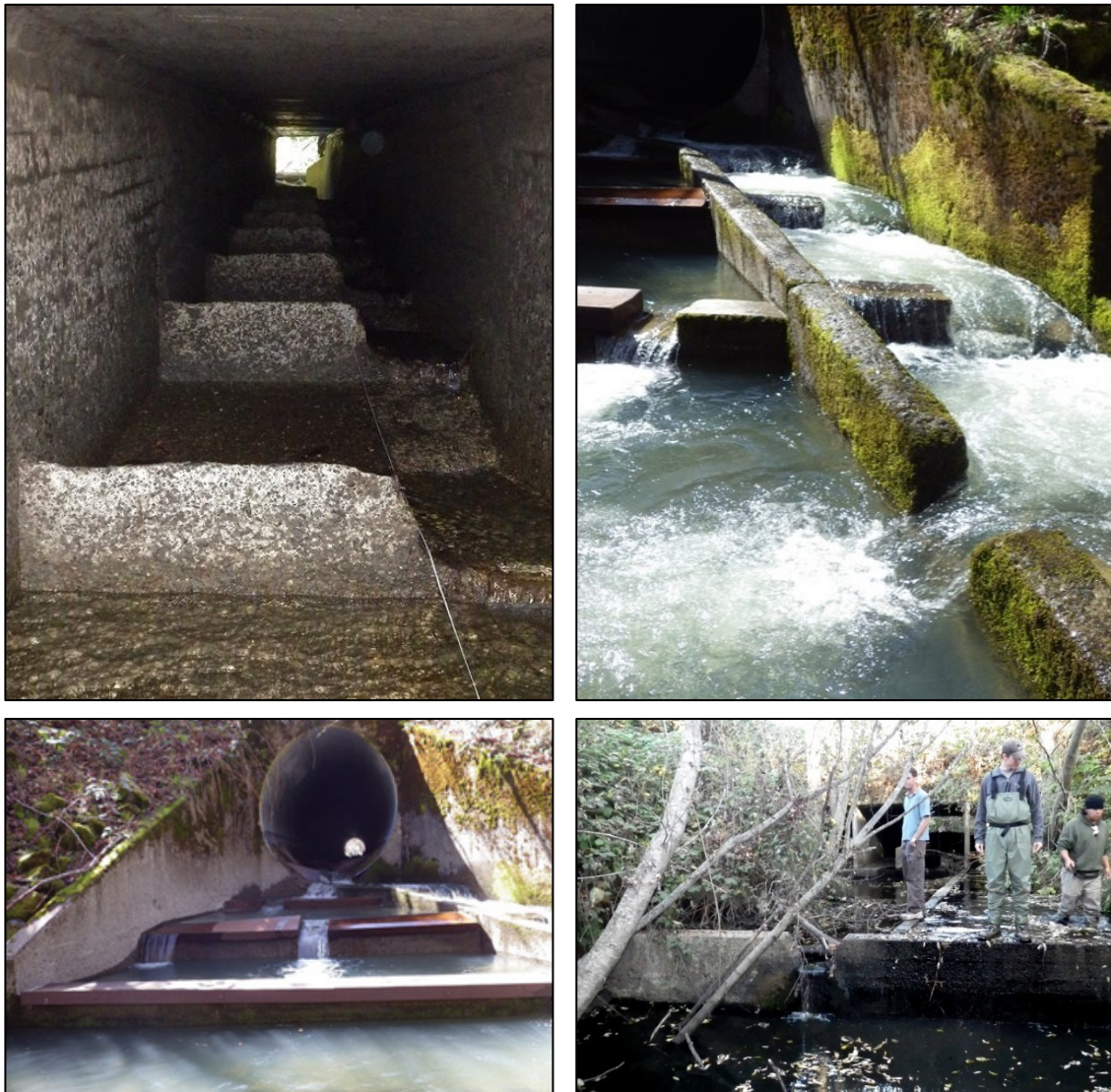
Figure 4. Examples of internal structures and modifications at road crossings that can impede lamprey passage in the Eel River basin, CA. Internal baffles with squared corners in undersized crossing (top left), step-pool fishways with square edges at outlet (top right and bottom left), and tailwater control weir with vertical drop and square edges (bottom right). Credit: Wiyot Tribe Natural Resources Department.
