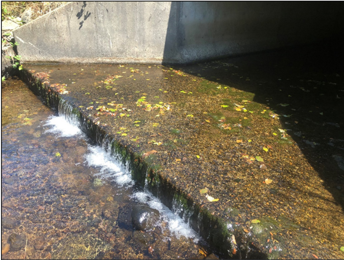
Figure 5. Example of culvert outlet apron with a vertical step at a crossing Munson Creek, Tillamook River watershed, Oregon. Credit: A. Gillette, ODOT.
