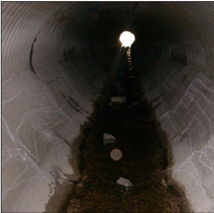
Figure 3. Pass Creek, post retrofit, showing smoothed concrete and “fish rocks” installed throughout invert of culvert to provide localized velocity reduction (left). Another example of “fish rocks” is shown (right) from a separate project, as the Pass Creek fish rocks were somewhat undersized for expected velocities.
