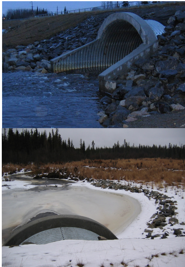
Figure 5. Beaver Creek inlet (top) and outlet plunge pool (bottom).
