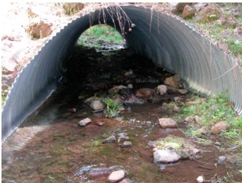
Fig. 16. Design Problem – Scour resistance of undersized streambed simulation material.
