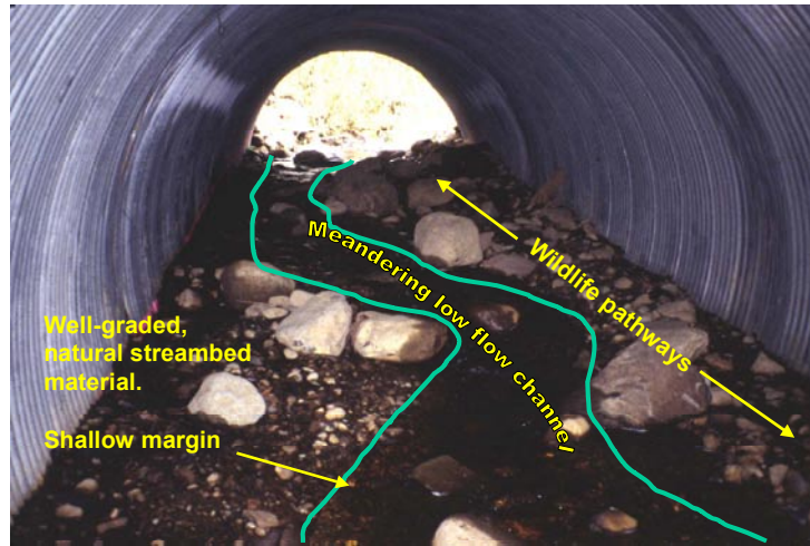
Fig. 13. A completed stream simulation project with bed simulation features.
