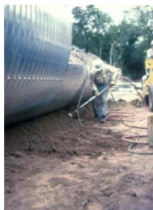
Fig. 7. Hand tamping bedding with a pneumatic tamper.
