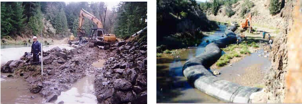
Fig. 3. Dewater only part of the stream to maintain aquatic organism passage.
