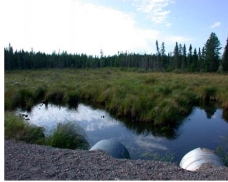
Fig. 1. Channel degradation downstream (left) and fig. 2 aggradation upstream (right) of a road crossing a wide floodplain on the Superior National Forest, Minnesota.
