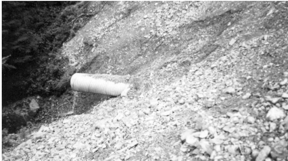
Fig. 7. Example of a shotgun culvert. Road #8576, Hoonah Ranger District, 1997.
