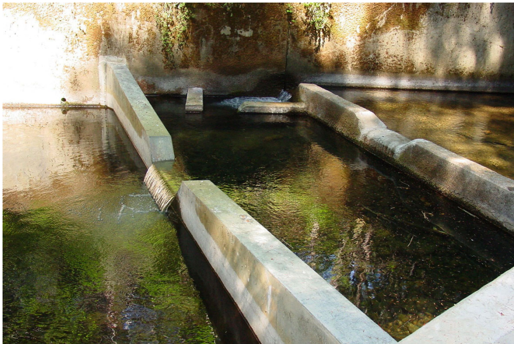
Figure 8.7. Notch weirs downstream of a culvert installation, acting to properly backwater the culvert, while maintaining manageable drops (United States Forest Service 2005).
