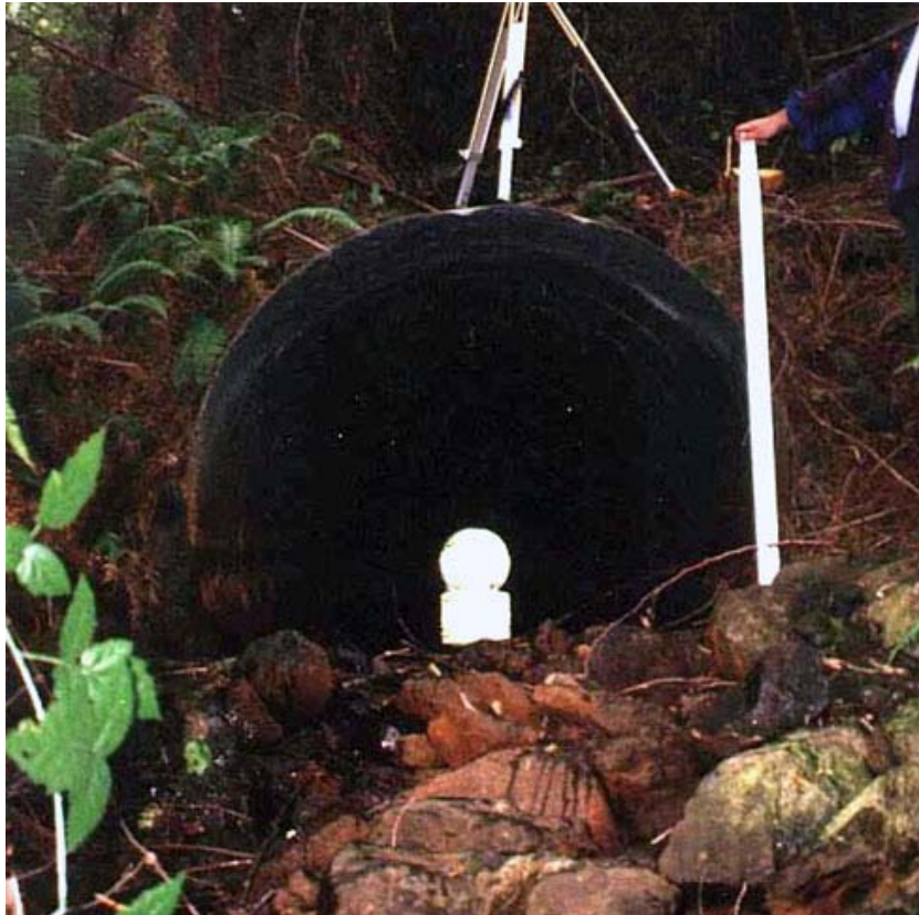
Figure 12.3. Pre Project Barrier Culvert (United States Forest Service 2006b)
