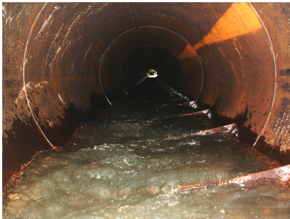
Figure 12.15. At high flows, baffles slow water velocities while producing minimal turbulence. Along the low side of the baffles, velocities are swift, improving passage of debris and sediment, while the high side of the baffle experiences slower velocities suitable for both adult and juvenile fish.
