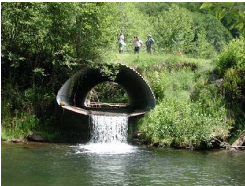
Figure 1.3. Downstream scour caused this culvert to become perched, as well as presenting a low flow barrier to fish passage (Furniss 2006).
