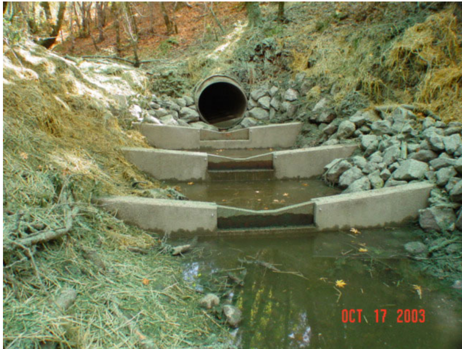
Figure 12.16. Culvert outlet after installation. Weirs below outlet were precast and lowered into place. Weirs were keyed into the bank roughly 2 ft and the contractor neglected to rock the left bank. The inspector failed to enforce this oversight.
