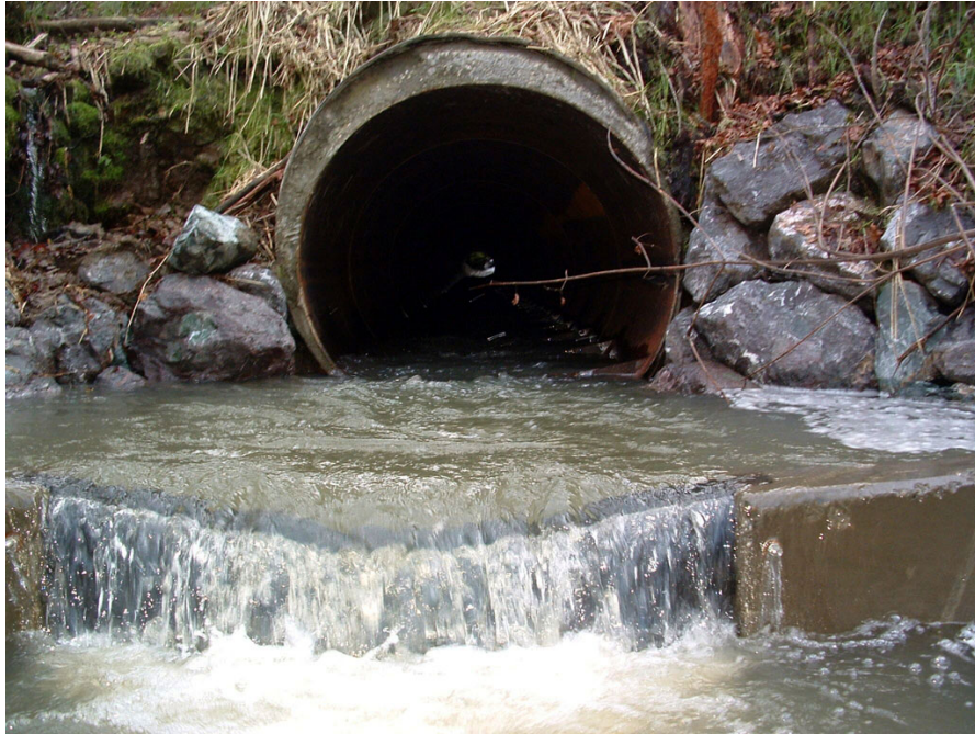
Figure 12.12. A 5 ft diameter welded steel pipe was inserted into the pre-existing culvert, concrete slurry was used to fill the gaps.
