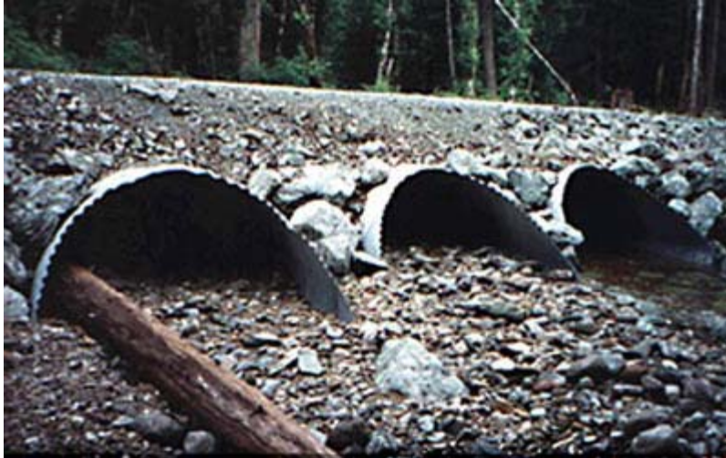
Figure 1.2. Multiple culvert installation located at a slope break where sediment is likely to deposit, creating a debris barrier. Flow is spread to thinly to allow fish passage (United States Forest Service 2006b).
