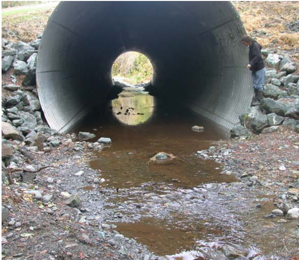
Figure 12.4. Replacement Culvert (United States Forest Service 2006b)
