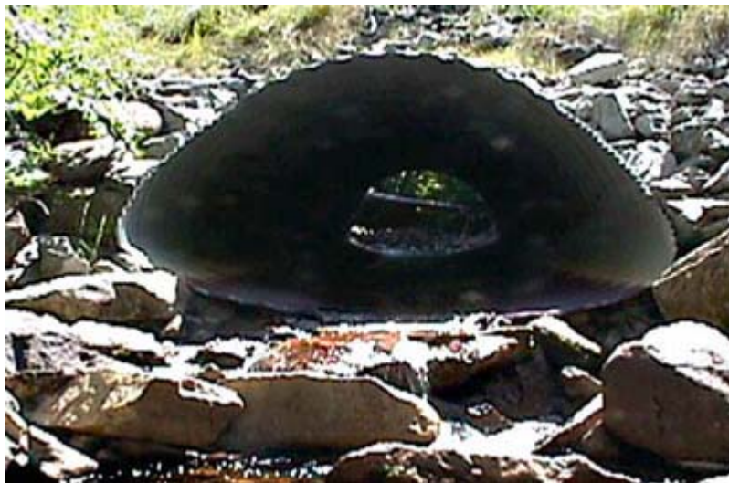
Figure 8.4. Downstream riprap will dissipate energy and reduce scour, but must be placed with fish utilization in mind. Riprap at this culvert exit effectively blocks fish passage (United States Forest Service 2005).
