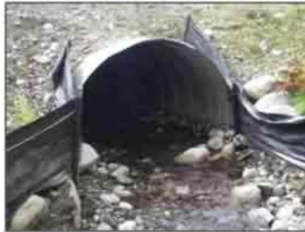
Embedded Circular Culverts
