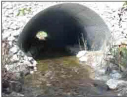
Embedded Circular Culverts
