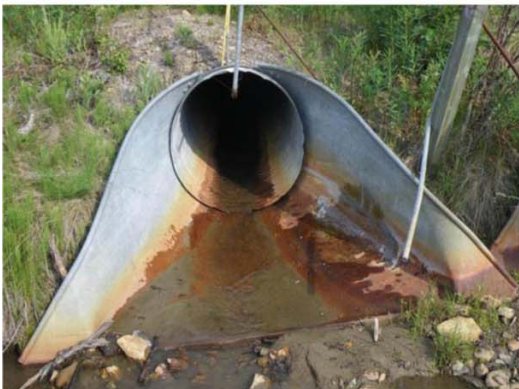
Flared Metal Apron Culvert
