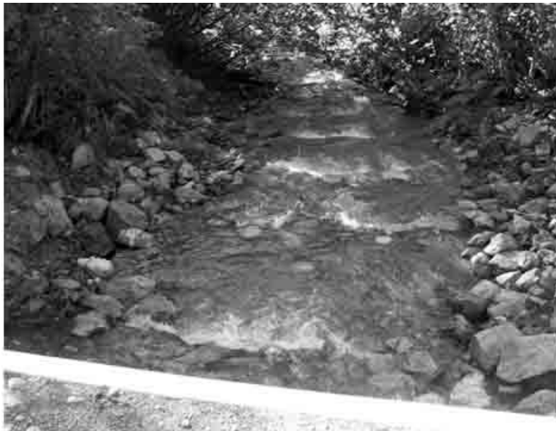
Figure 25b.—Looking downstream at a series of step pools constructed as part of a culvert replacement project.
