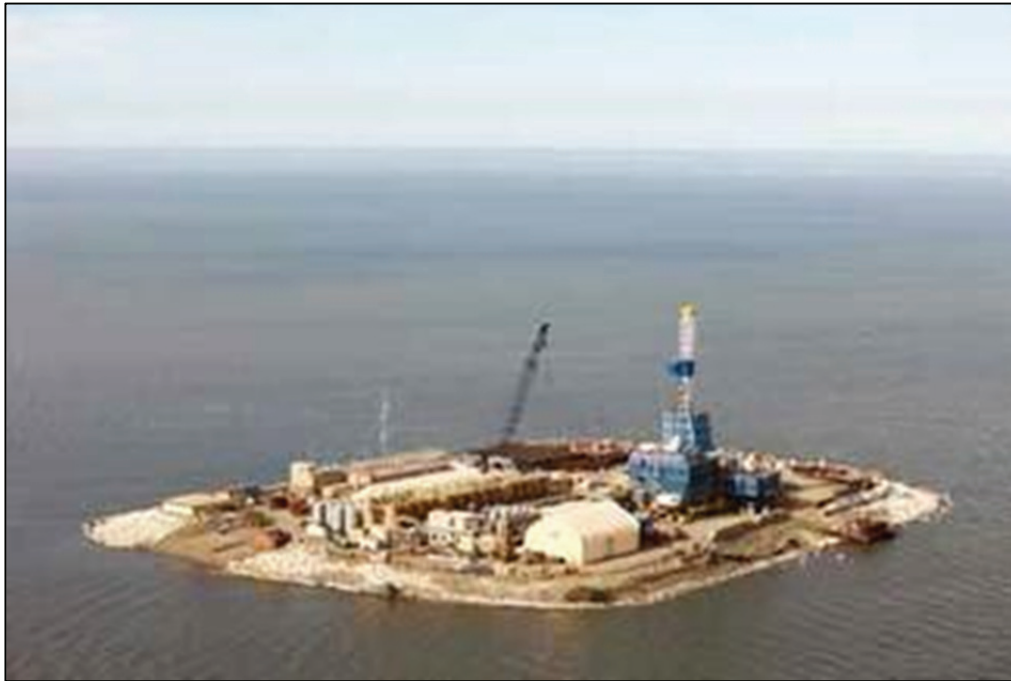
Figure 3.3-17 BP, Liberty exploratory drilling site.
