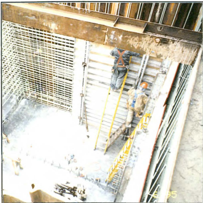
Installing rebar and formwork for seawater well walls.
