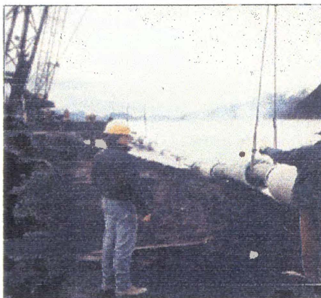
Placement of seawater intake line.
