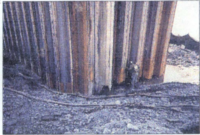
Sheetpile damage caused by underground obstruction.
