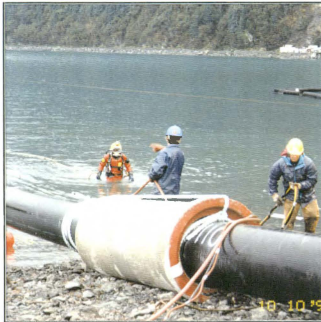
Concrete anchor around seawater intake line.
