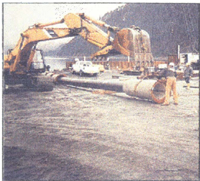
Installing concrete anchors on seawater intake line.
