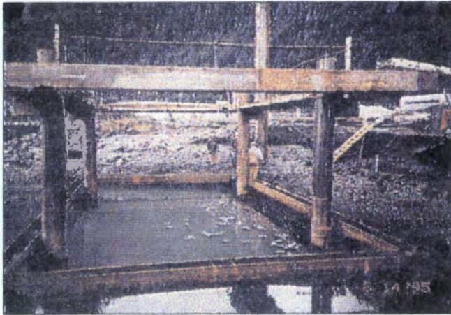
Seawater well sheetpile template in place.
