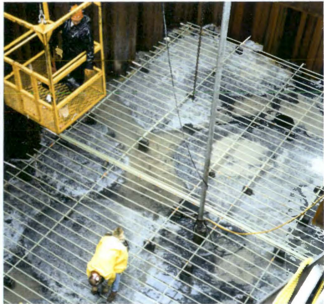
Placing seawater well slab epoxy coated reinforcing bars.
