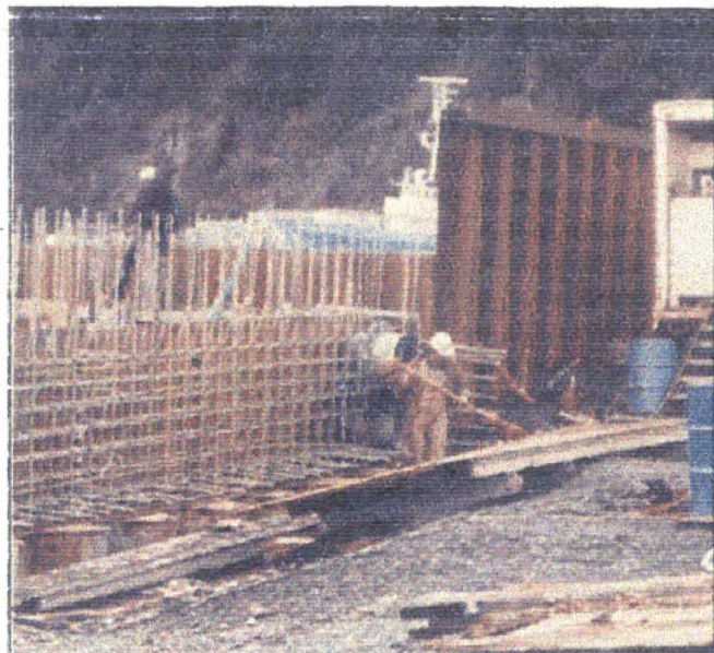
Installing rebar and formwork for seawater well walls.
