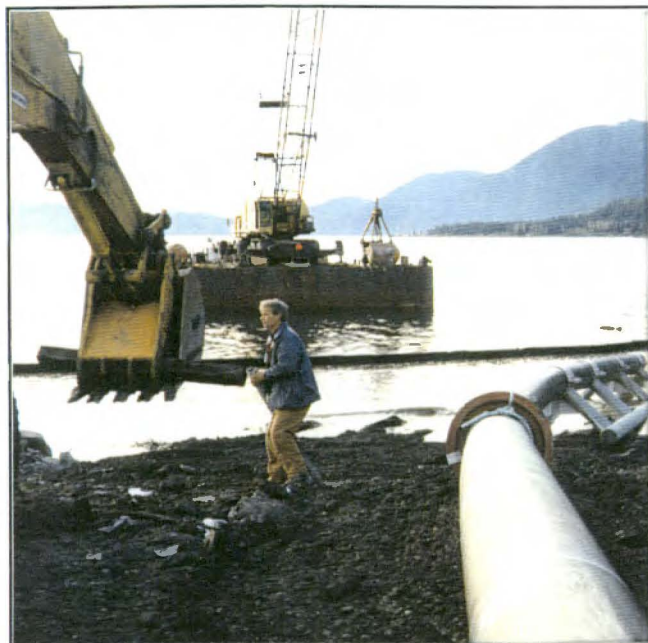
Preparing seawater intake pipe for water placement.
