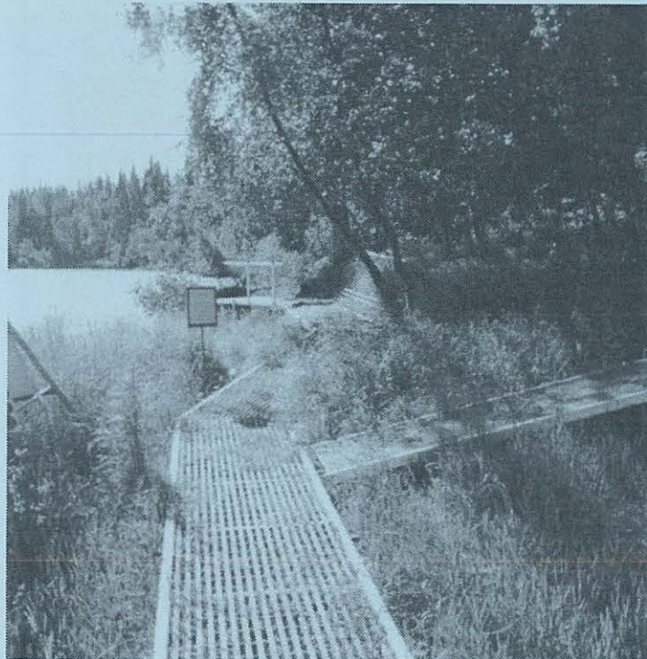
Endicott Sonar site elevated gratewalk.
