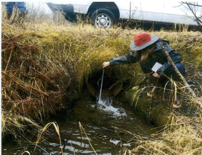
Photo 1: Perched culvert on a Battery Creek tributary
