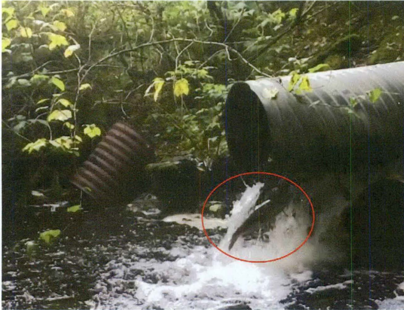
Photo 4: A coho salmon failing to pass a perched culvert at Boy Scout Lake outlet
