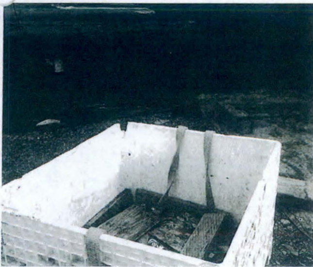
PHOTO 7: DEBRIS BIN, TARP BMPs
