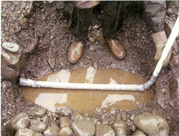
Figure 6: Photo of a 1.0 m trench with the manifold placed parallel to the shoreline before refilling the trench. A more rigid system is being proposed for the delivery of chemicals in this study.
