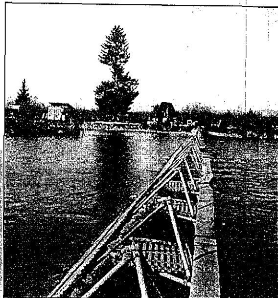
The adult weir at the Coghill River creates a barrier for sockeyes returning to the system. They are allowed to pass through a portion of the barrier, at which time they are individually counted by ADF&G field staff. (Photo by Grant Bremer)
