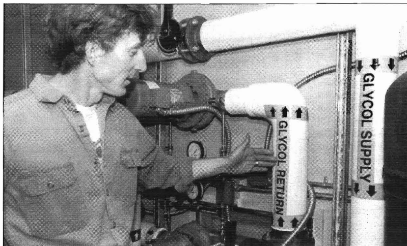
Chuck Pratt, Assistant Manager at AFK hatchery, points out the heat exchange system in the new boiler unit. Photo by L. J. Evans
