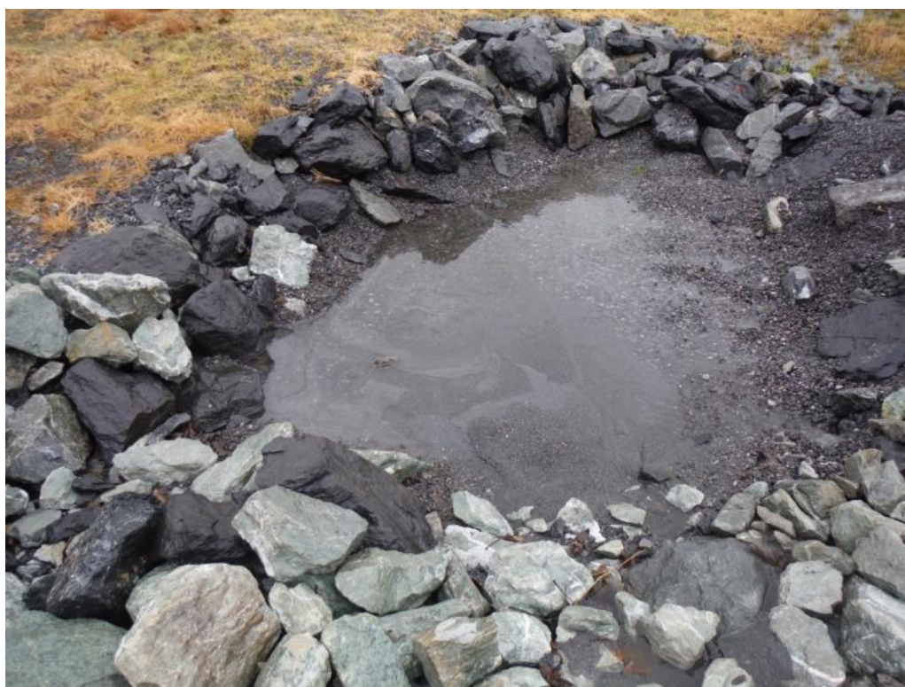
Sheen on water surface in Odiak Pond snow storage sediment trap from parking lot runoff. February 2016
