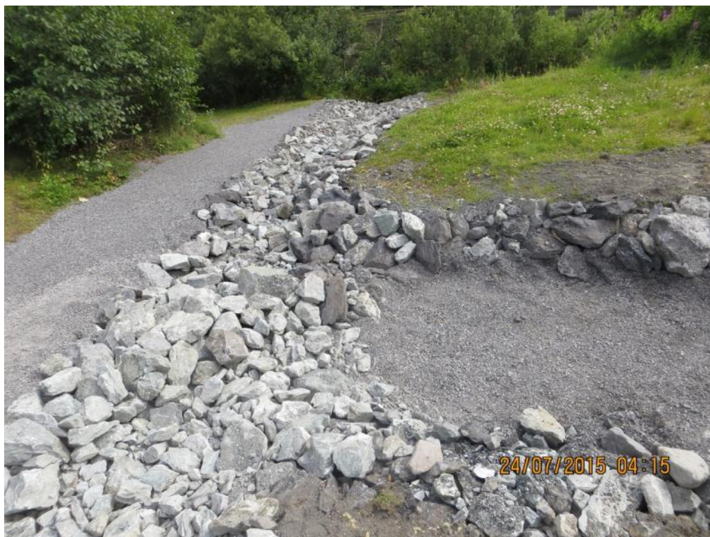
Re-constructed foot and vehicle access path, rip rap drainage ditch to prevent erosion of gravel and fine sediment, and sediment trap basin. July 2015.
