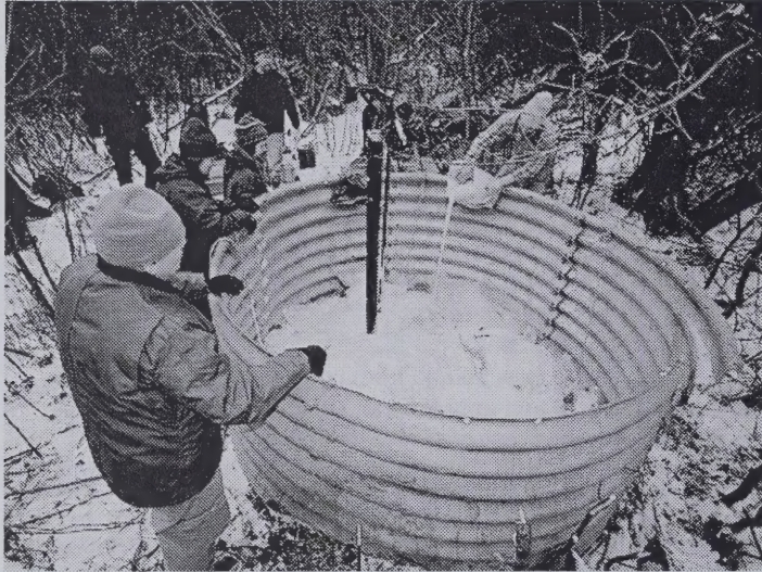
Pouring foam as crew watches — about 3 feet more to go.
