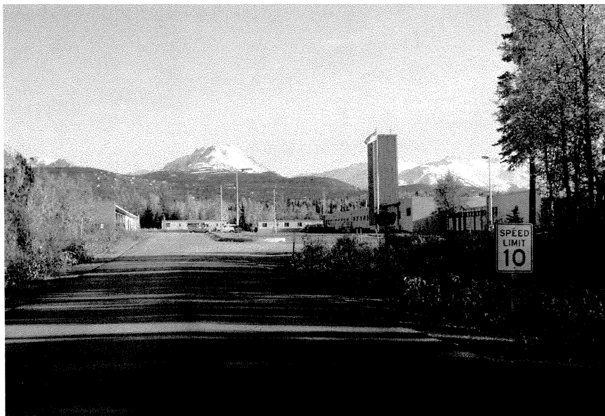
Figure 28. Developed area, Campbell Tract Facility.
