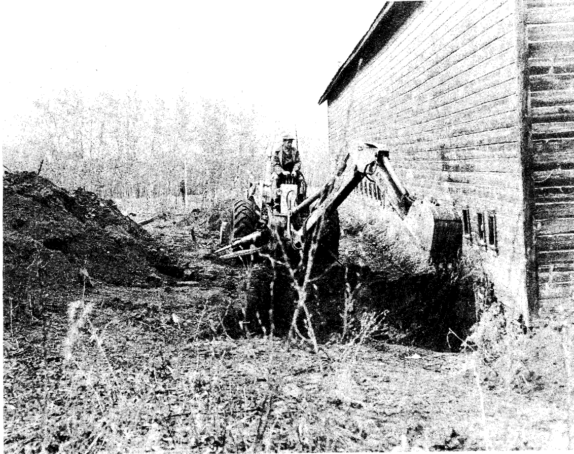
Fig. 70. Stabilization trenching on the stables' north side.
