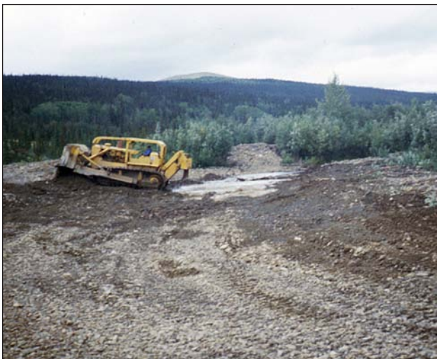
Figure 7. The bulldozer constructed the channel using short, almost level grading to deepen the pilot channel.
