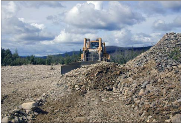
Figure 6. After filling the ponds, the bulldozer then graded the floodplain as flat as possible.
