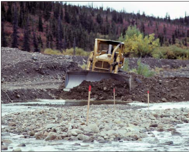
Figure 5. The initial step in reclamation was to fill the settling ponds with the dozer, using the material from the surrounding tailings piles.
