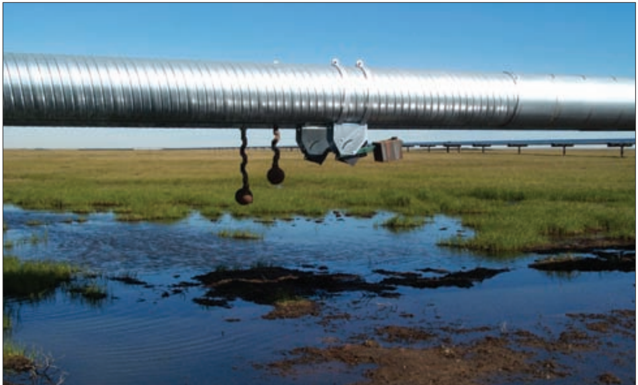
Figure C-2. Kuparuk DS-2L pipeline elevated to 1.5-m minimum height and showing older spherical style and newer “potato-masher” style of vibration oscillation dampeners, and reflectivity of standard sheathing. Photo by B. Lawhead, ABR, Inc. Copyright ConocoPhillips Alaska, Inc.
