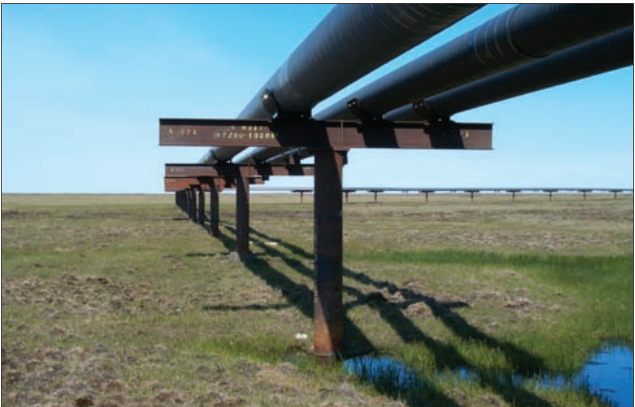
Figure C-3. Pipelines with nonreflective sheathing and elevated to a minimum height of 2.1 m, constructed in winter 2001–2002, Kuparuk DS-3S project, northern Alaska. Photos by B. Lawhead, ABR, Inc. Copyright ConocoPhillips Alaska, Inc.
