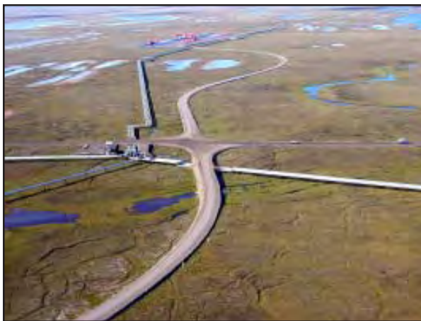
Figure 3. Gravel roads in Prudhoe Bay area (2002).
