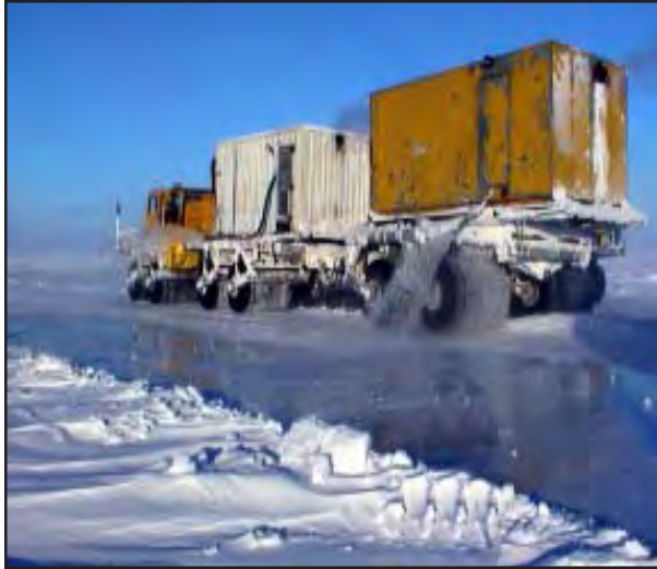
Figure 7. Water added to ice road layer.
