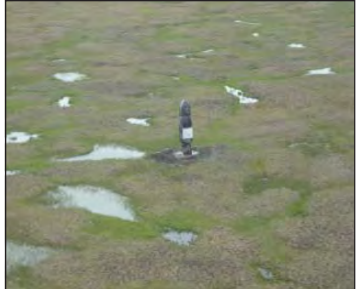
Figures 22 and 23. Puviaq test well and ice drill pad in March 2003 (left) and in July 2003 with only well head remaining (right).
