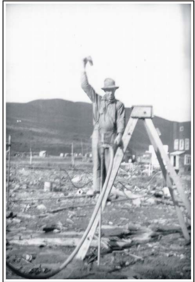
Figure 55. Barnett Photograph #53: An unidentified employee of the Matheson Dredge driving points in Flat.
