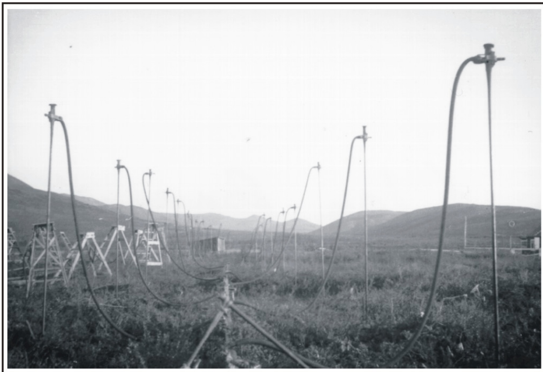
Figure 36. Barnett Photograph #34: Driving points for the Donnelley dredging operation, Otter Creek.
