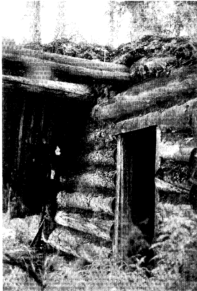
7/31/82 Side/front of Cabin #6 showing roof decay and log fallen across it.
