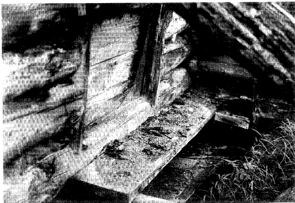
7/29/82 Inside of Cabin #1 showing shelves and window.
