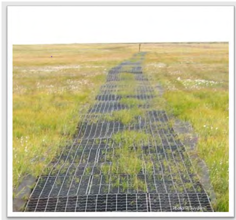
Photo 6: Example of geogrid application mitigating anthropogenically-derived surface water in Utqiagvik. Photo Credit: NSB Website- Robert Suydam
