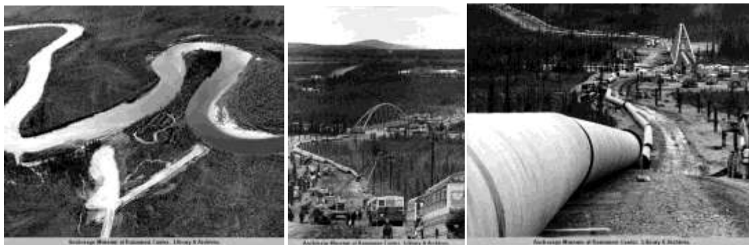
Figure 30. Construction work for the bridge over the Gulkana River during the pipeline construction in 1976 (source: Alaska Virtual Library and Digital Archives).
