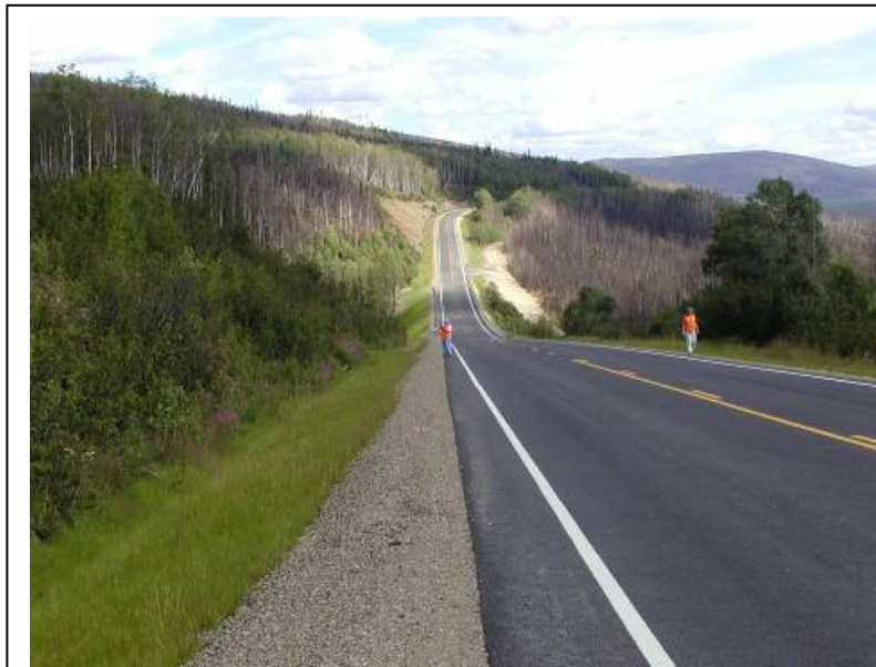
Figure 7. Recent road construction work near Davidson Ditch.
