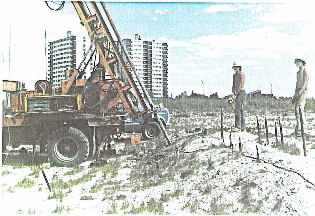
FIELD DRILLING - GRAVEL SECTION
