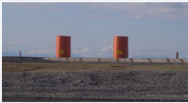
Existing capped wells at the Central Pad
