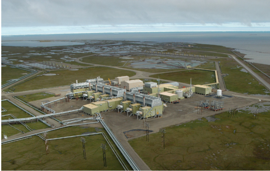
Photo courtesy of BP Prudhoe Bay Central Compression Plant
