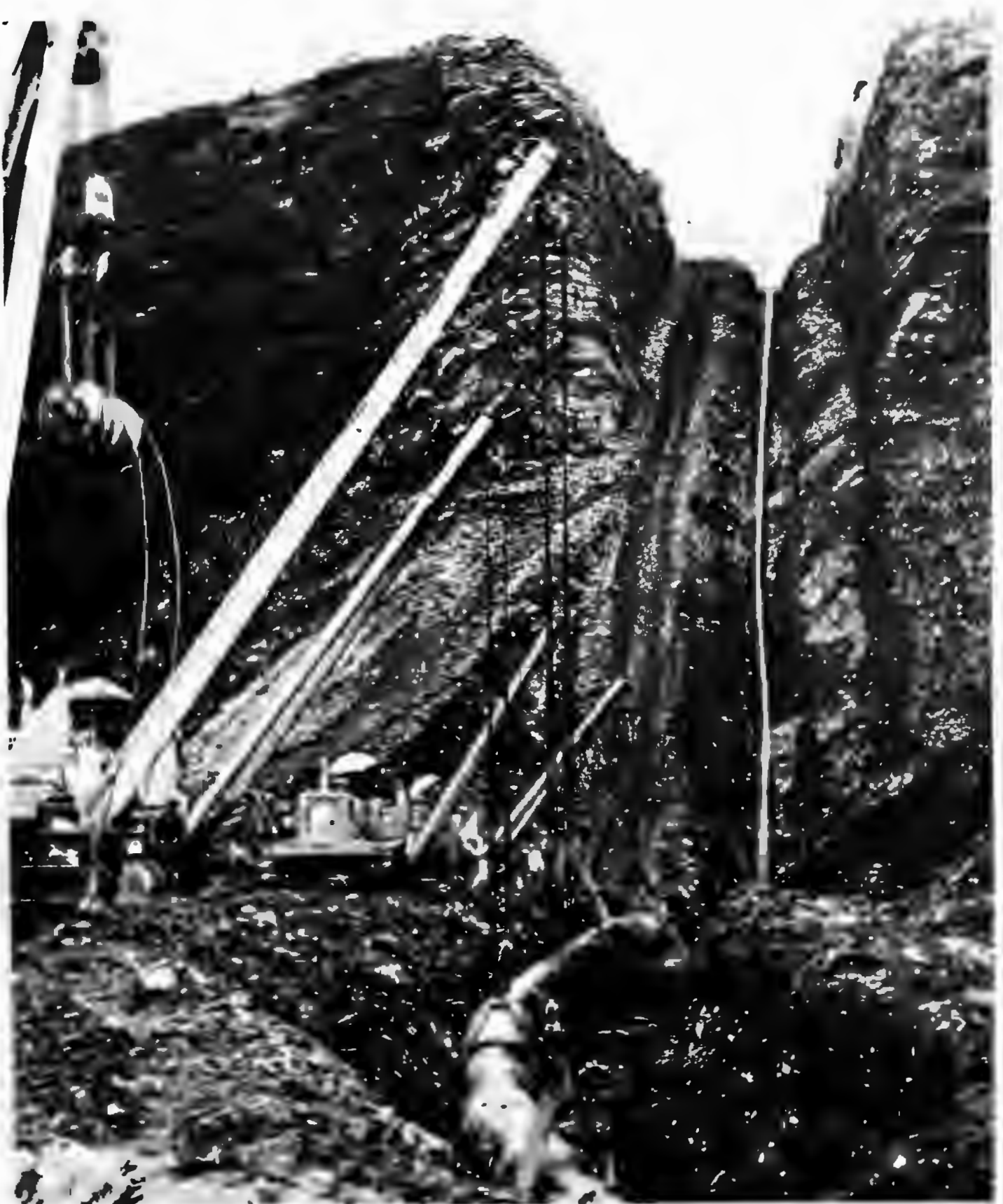
Pipe being lowered into trench on trans-Alaska oil pipeline. Similar techniques are proposed for natural gas pipeline construction (Alaska)
