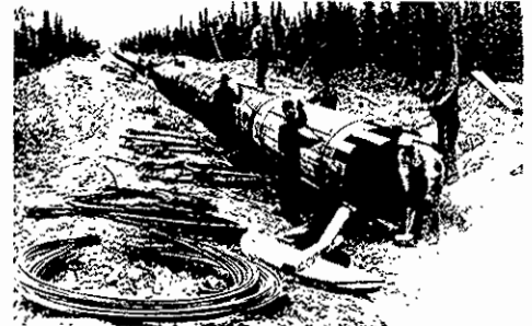
A wood-stave pipe used to carry water to Klondike placer mines.
