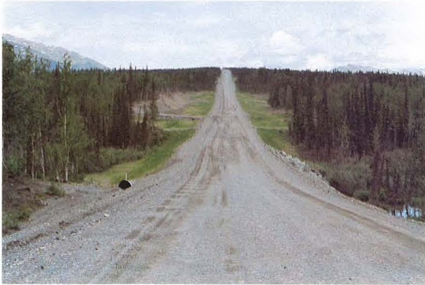
Plate 15. A portion of the Haul Road constructed through spruce-deciduous woodland (HMQ) in A.S. 97, Section 4. View is north. Note new growth on the cut and fill slopes from revegetation with grasses. JFWAT photo 817-3 by the author; June, 1977.
