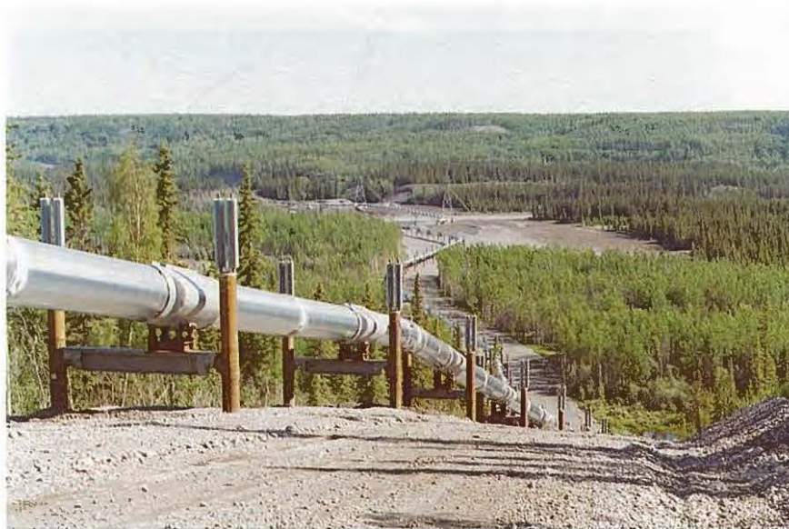
Plate 18. A section of above-ground (elevated) pipeline constructed in spruce-deciduous woodland (HMQ) in A.S. 21, Section 1. A staging area on the south bank of the Tazlina River can be seen in the center of the photo. Note the thermal radiators used to dissipate heat atop the vertical support members (VSM's). The 48 inch pipe is encased in a galvanized covering and attached to steel, sliding "shoes" which rest upon cross members. JFWAT photo 833-7 by the author; June, 1977.
