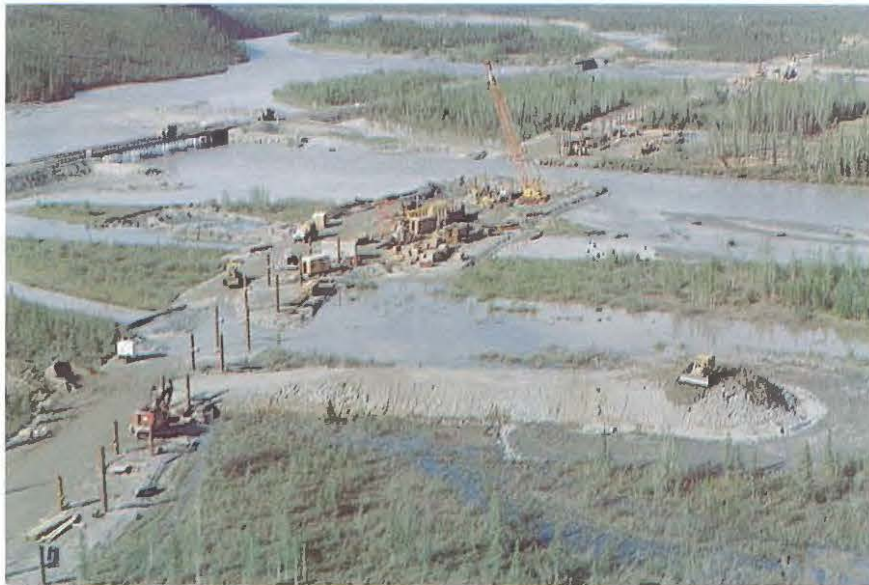
Plate 24. Spur dike construction (dozer on "nose" of dike) and river-crossing staging area on the Hammond River, A.S. 101, Section 5. The pipeline crosses the Middle Fork Koyukuk River in the upper right corner of the photo. View is north. Haul Road is to the west of the pipeline. JFWAT photo 545-10 by C. Burger; June, 1976.
