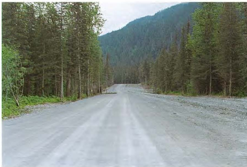
Plate 17. A section of work pad and completed below-ground pipeline through coastal forest (MQ) in A.S. 2, Section 1. The pipeline is buried on the right side with the driving surface on the left. JFWAT photo 832-1 by the author; June 1977.
