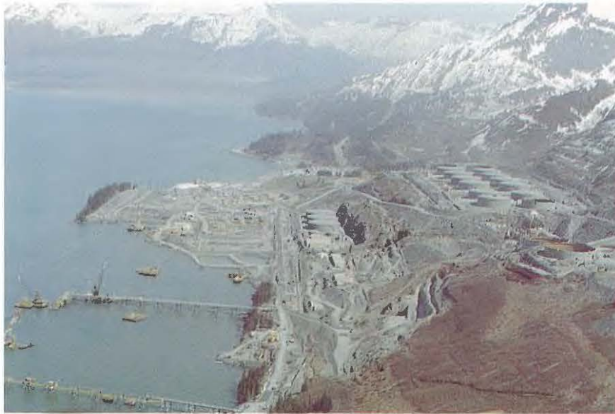
Plate 23. The Valdez Terminal, constructed in coastal forest (MQ) and shrub thickets (HMQ), adjacent to Valdez Arm in Prince William Sound. Oil storage tanks can be seen on the uplands with loading docks for the oil tankers extending into saltwater. JFWAT photo 551-2 by J. Gustafson; June, 1976.
