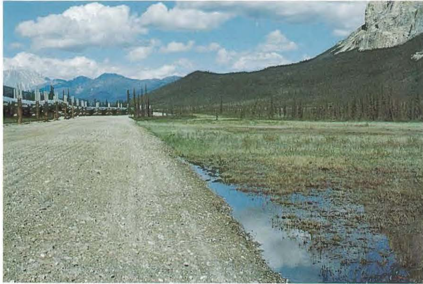
Plate 19. Work pad and elevated pipeline built through wetlands (HQ) in A.S. 103, Section 5. View is north. Cross-drainage is from east to west; note ponding on right side of pad. JFWAT photo 817-6 by the author, June, 1977.
