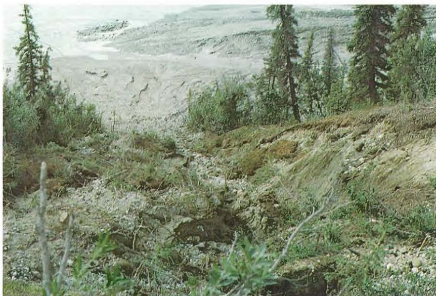
Plate 14. Results of thermal erosion downslope of a Haul Road culvert (station #2307 + 92) in A.S. 103, Section 5. Material eroded directly into a side channel of the Middle Fork Koyukuk River. This type of erosion occurred at several locations in A.S. 102, 103, and 105. JFWAT photo 578-18 by J. Gustafson; June, 1976.
