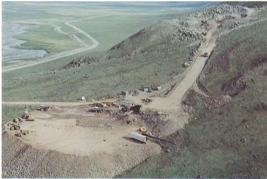
Plate 31. M.S. 112-3.1 and a disposal area built in tussock tundra (MQ) and alpine tundra (LMQ) on the north side of the Brooks Range, A.S. 112, Section 5. View is north. An access road leads to site. Work pad lies between the Atigun River and the Haul Road in photo background. JFWAT photo 577-9 by J. Gustafson; June, 1976.
