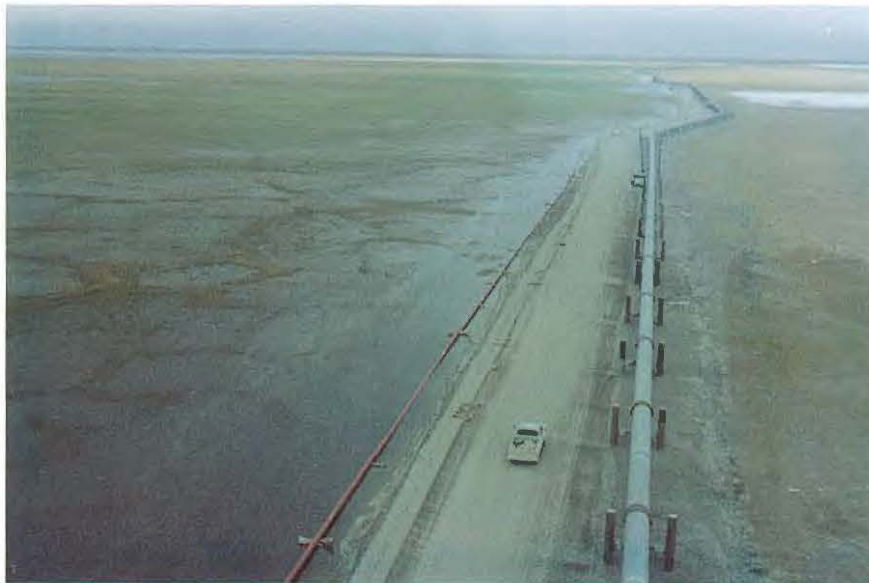
Plate 20. A section of work pad through wet-meadow tundra (HQ) in A.S. 137, Section 6. View is north. The fuel gasline can be seen on the west side of the pad with the 48" pipeline on the right side. Both segments of pipe are resting on wooden cribs prior to installation. Note ponding on west side of pad throughout photo. JFWAT photo 652-30 by M. Buckley; June, 1976.
