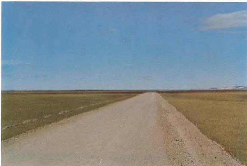
Plate 16. A portion of the Haul Road through wet-meadow tundra (HQ) in A.S. 130, Section 6. View is north. The narrow line of ditch spoil paralleling the Haul Road on the west side is from the burial of a natural gas, fuel line which runs from Pump Station 1 to Pump Station 4. JFWAT photo 844-4 by E. Westman; July 1977.
