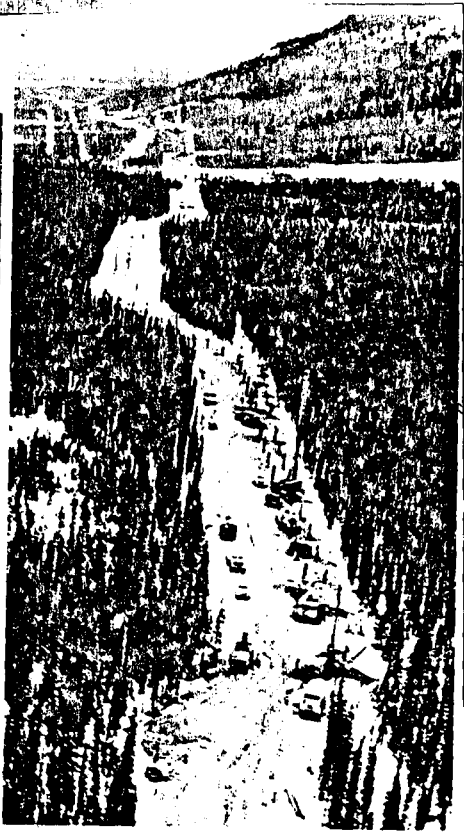
A Zig-zag right-of-way across the wilderness illustrates special design employed on elevated sections. In foreground, three different makes of drill rigs dig holes for the VSM's. — Courtesy Standard Oil Co. (Ohio)
