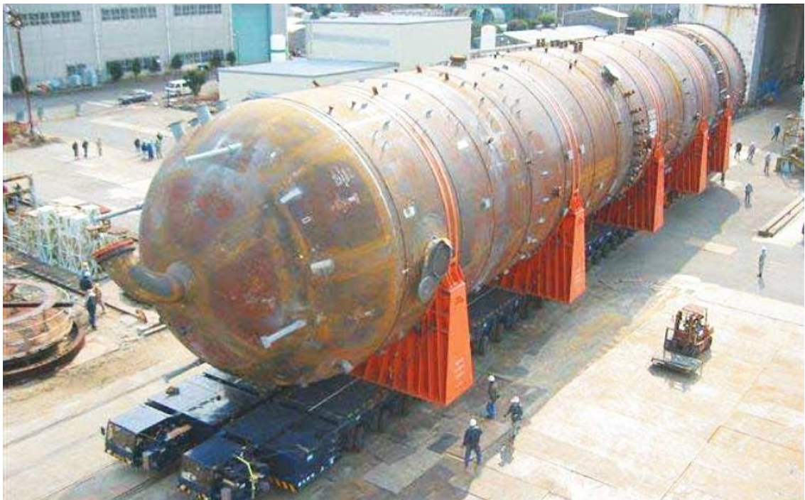
Figure 7-3: Transport of one 17,000 bbl/day Slurry-Phase FT Reactor [8]
