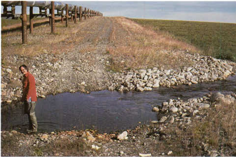
Plate 5 Typical low water crossing with armored banks, widened pool at vehicle ford and constricted outlet which helps prevent blockage at low flow (Polygon Creek, MP. 99).
