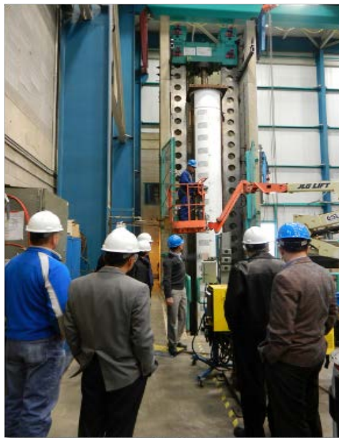
The Alaska Pipeline Project recently began testing pipe in Canada for use in the Alaska natural gas pipeline. Photo courtesy of the Alaska Gas Pipeline Project Office.
