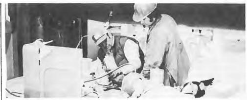
Foothills and contractor personnel monitor testing of high-pressure discharge piping at Richmound compressor station.
