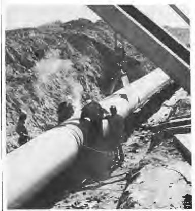
The final tie-in weld, completed on August 17 south of Beiseker, Alberta, wraps up construction on the Eastern Leg of the Alaska Highway gas pipeline in Canada.
