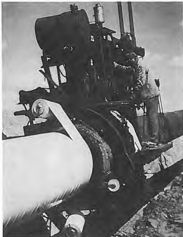
A wrapping machine cleans the pipe, coats it with tar paint, and wraps it with polyethylene tape to protect the pipe from corrosion.
