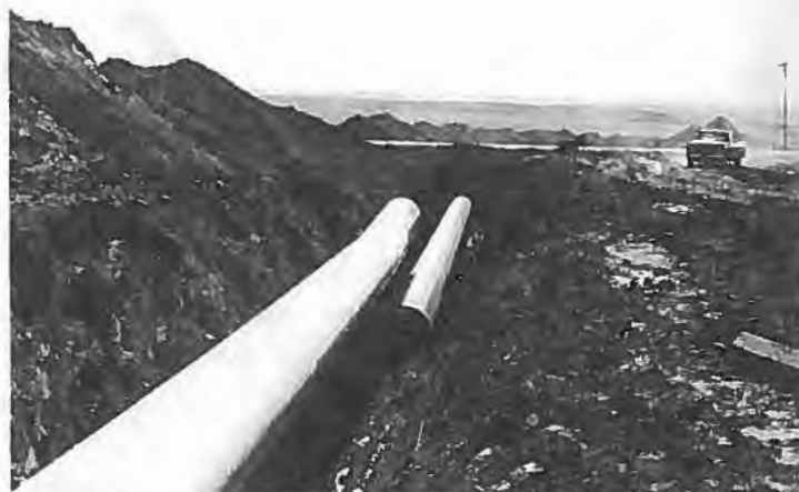
Gaps in the pipeline which require tying-in are left at road, railroad, water crossings and game/farm animal crossings. At tie-ins extra pipe is cut off, the edges bevelled, welds are made and protective tape is then applied.
