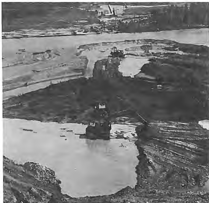
Ditching the Red Deer river crossing in Alberta took about 10 days, using a 245 Caterpillar backhoe. A total of 271 m (889 ft.) of pipe, coated with concrete, was pulled through the river, laid in the ditch and buried with three m (10 ft.) of cover.
