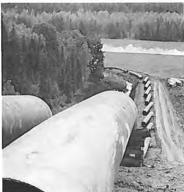
The right-of-way is cleared, graded and ditched and the pipe strung alongside and bent to follow the rolling terrain near Olds, Alberta. Pipe bends are achieved through careful calculation and by a series of short pulls with a hydraulic bending machine.
