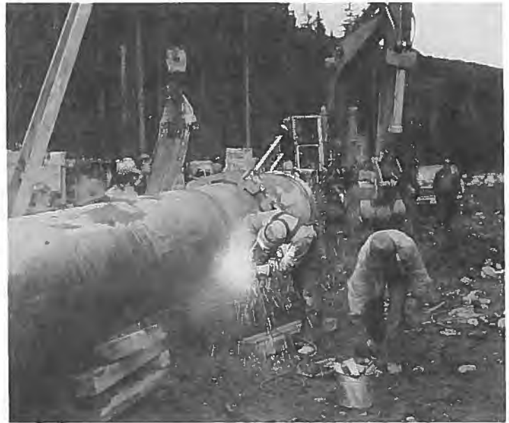
With manual or stick welding, an electric arc melts and fuses the metal of the pipe ends with the metal of the stick electrode used by the welder. Completed welds are reinforced by an additional four or five welds.
