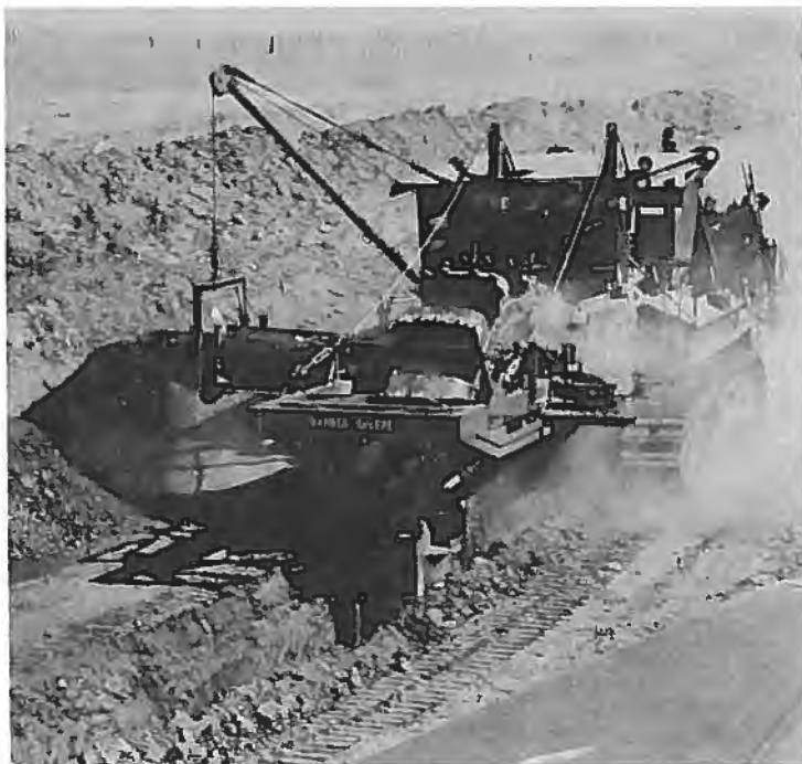
A ditcher capable of digging a trench three m (10 ft.) deep and two m (6.5 ft.) wide is used to allow for a minimum of 0.8 m (three ft.) of cover over the pipe.
