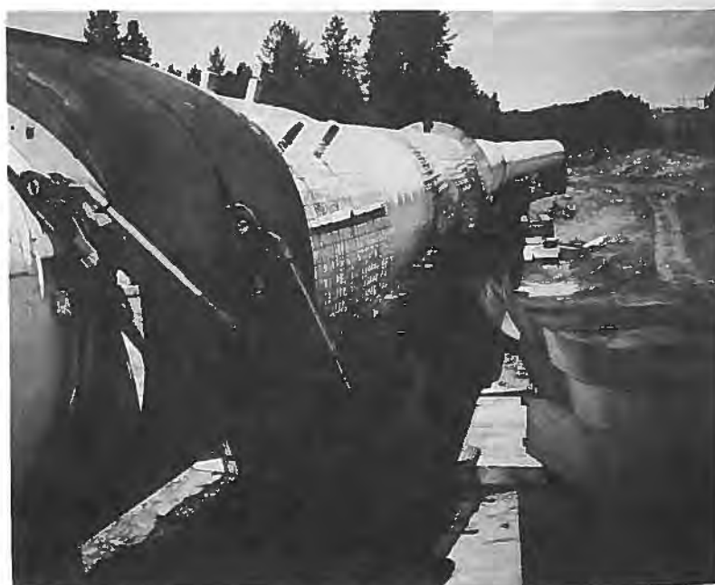
In preparation for a river crossing, the pipe is coated with concrete to weight it down in the riverbed.
