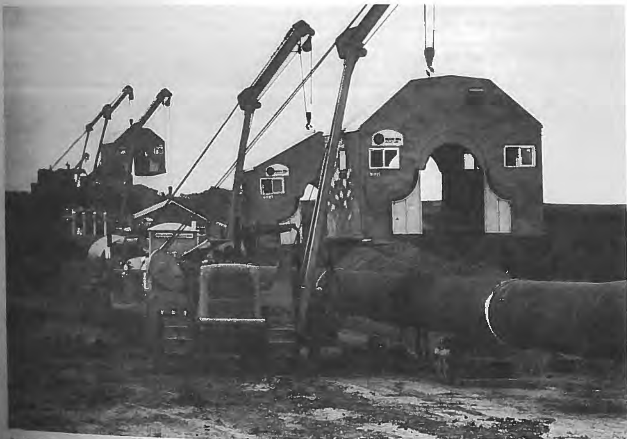
Automatic welders used on major spreads move along the pipe. The huts housing them permit welding to continue despite variable weather conditions. Following welding, the weld joints are covered with film negatives and an x-ray machine travels through the pipe and photographs each weld to check for imperfections.
