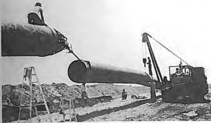
Accurate alignment of pipe for the stringer bead or first weld is critical in producing a sound weld. The edge of the pipe end must be machine-bevelled and the pipe ends properly spaced.
