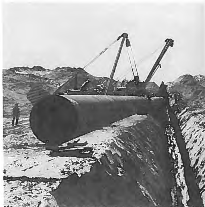
The V-shaped ditchline in the Great Sand Hills area of Saskatchewan is sloped to prevent the fine sand walls from caving in.
