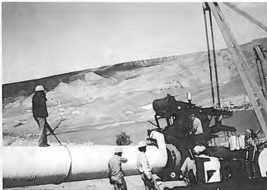
A crew member - known as a "jeep" - walks along the pipe behind the wrapping machine with an electronic circular hoop to detect faults in the tape.
