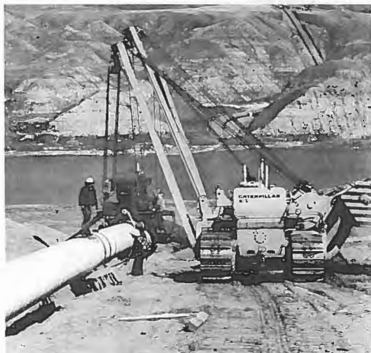
Pipe is often wrapped and lowered into the ditch with sideboom tractors in a continuous motion, called cradling-in. This reduces the amount of pipe handling by eliminating the steps of placing the pipe onto skids and then picking it up later for lowering-in.
