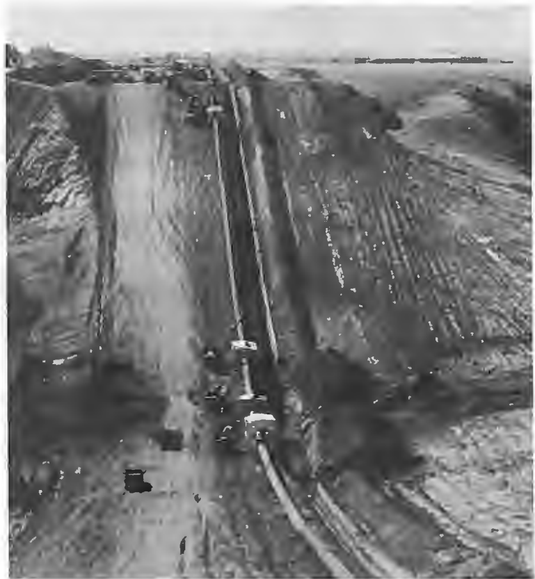
Automatic welders move down the 45 m (140 ft.)-deep west bank of Irishman's Coulee, Alberta.
