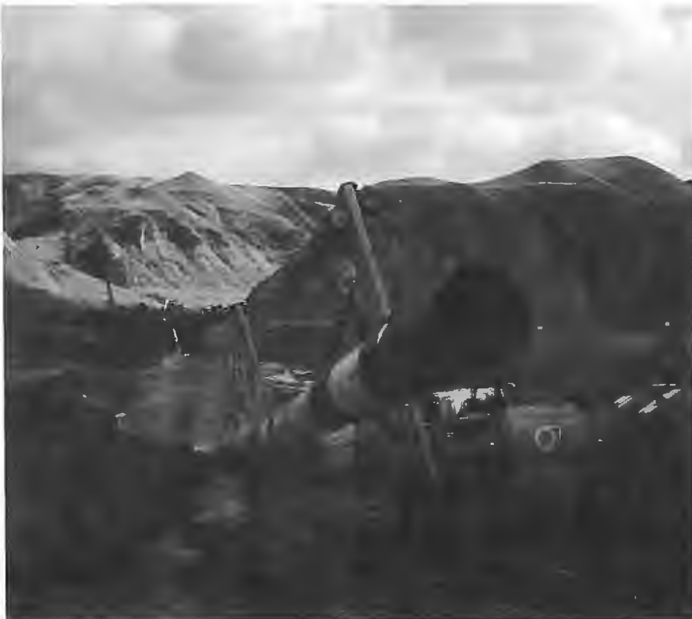
View from the west bank of the South Saskatchewan River. The pull is almost complete as the end of the pipe attached to the cables surfaces on the opposite shore.
