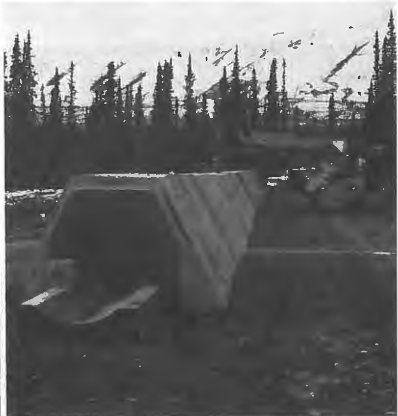
Abovegrade pipeline construction tested at Quill Creek facility in Yukon. Pipe installed on insulated workpad in gravel embankment mode (left) and concrete restrained mode (right).
