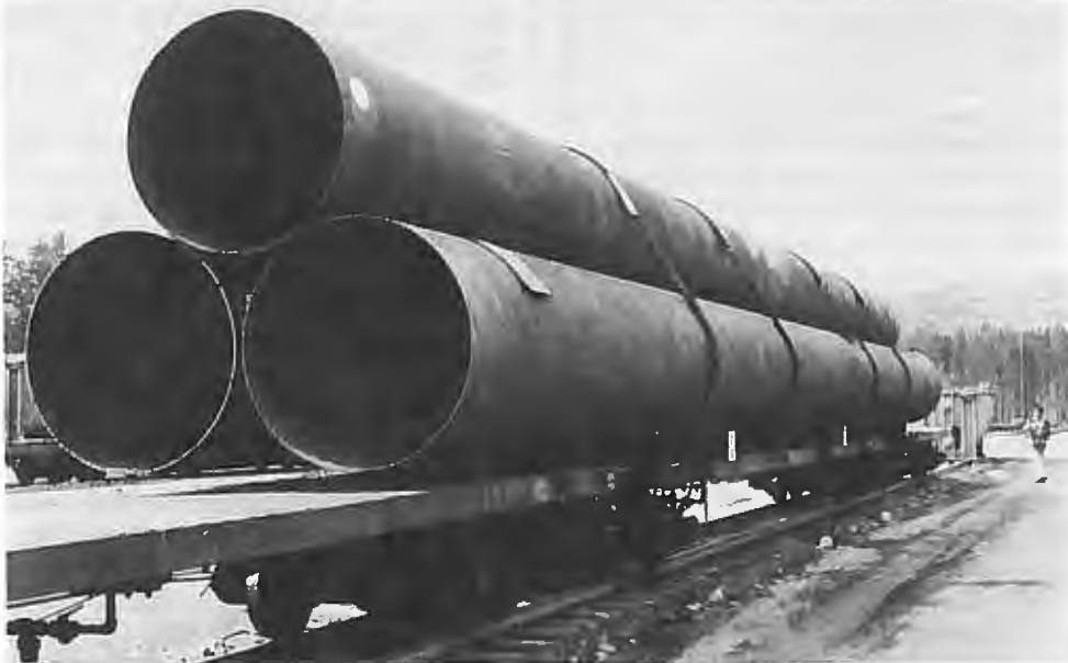
Three joints of 1,219 (56 in.) diameter pipe were hauled by the Whitepass & Yukon Railway in a successful test run from the port of Skagway, Alaska, to Whitehorse. The 25 metre (80 ft.) pipe lengths, weighing 11 tonnes, were strapped to a specially prepared flatcar and overhung on two adjoining cars. The experiment was conducted to determine how well the narrow gauge railroad could move long joints of pipe for the Alaska Highway gas pipeline.
