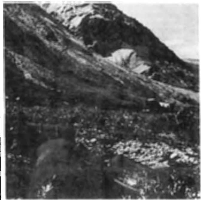
Remnants of Pump Station No. 4, 100 km (112 mi.) southwest of Norman Wells. The camp yard which was originally denuded of vegetation now has a dense willow shrub cover.
