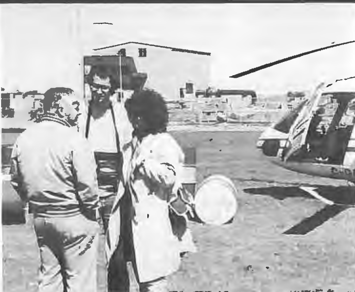
Senior Surveillance Officer Jim Wallace (left) shows construction underway at Jenner, Alberta compressor station to visiting Swedish journalists. A natural gas pipeline, the first in Sweden, is planned for construction.
