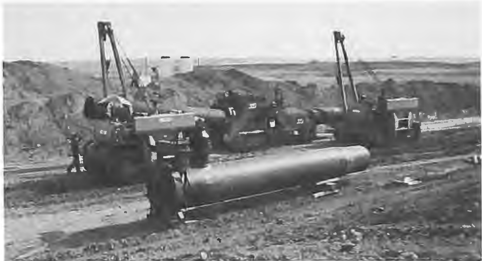
Pipe bending operations near Standard, Alberta
