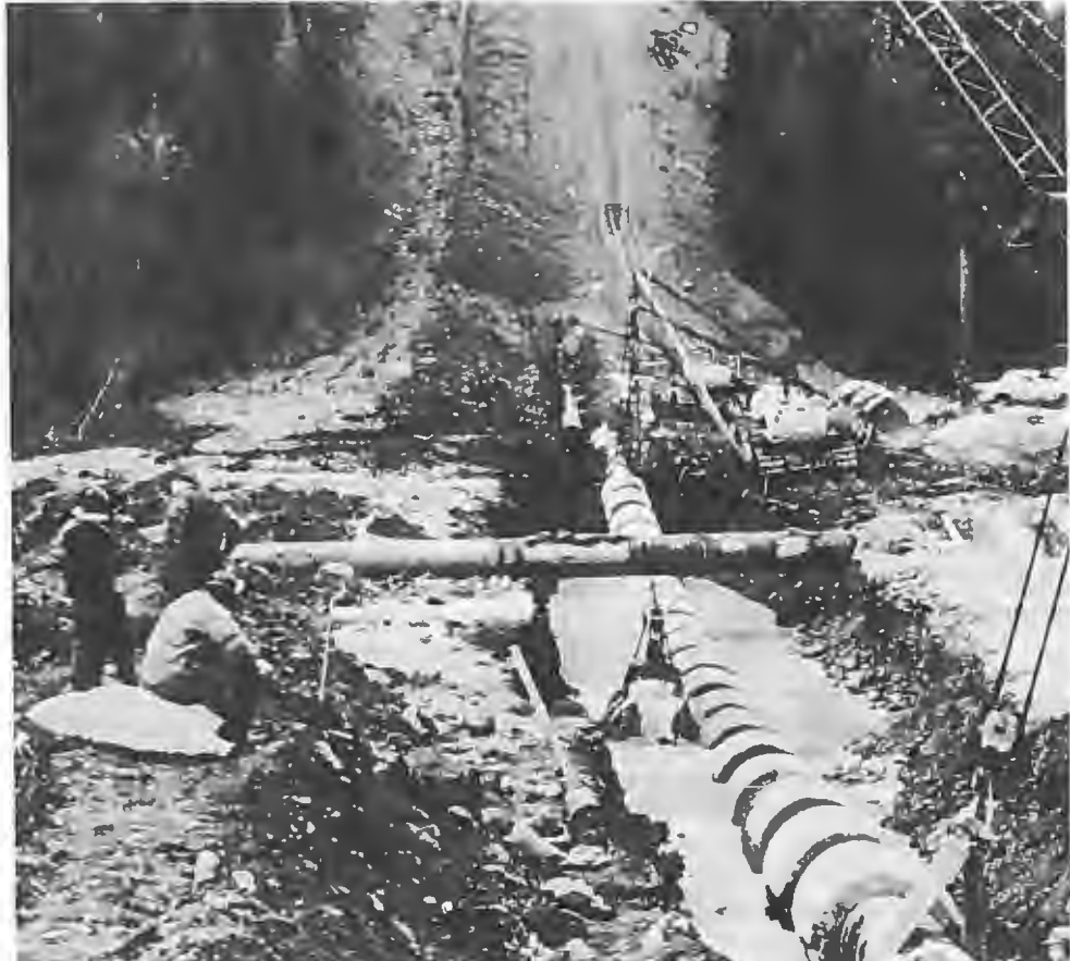
Flumed crossing of TeePee Creek in southern B.C.
