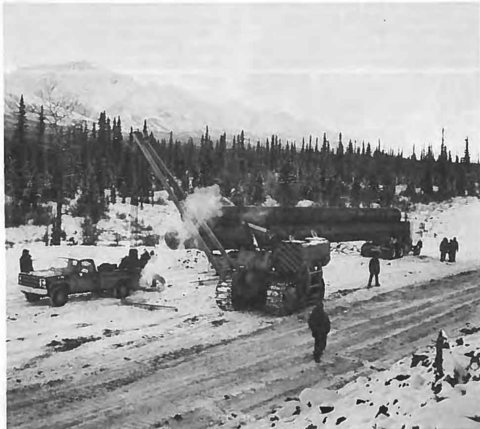
Crew unloads 80-foot lengths of pipe at Quill Creek test site.
